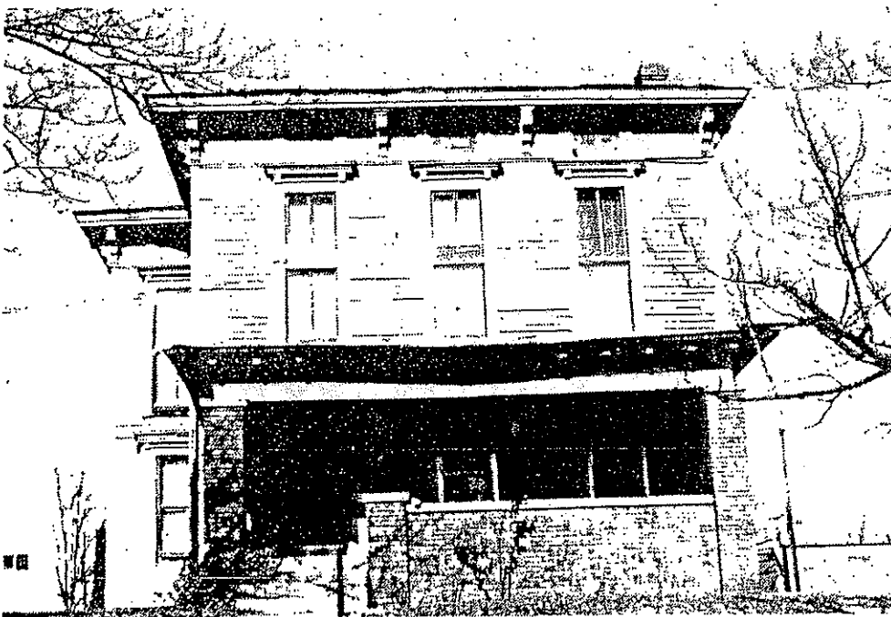
Photo 23 - Old home with significant architectural character in need of rehabilitation.
