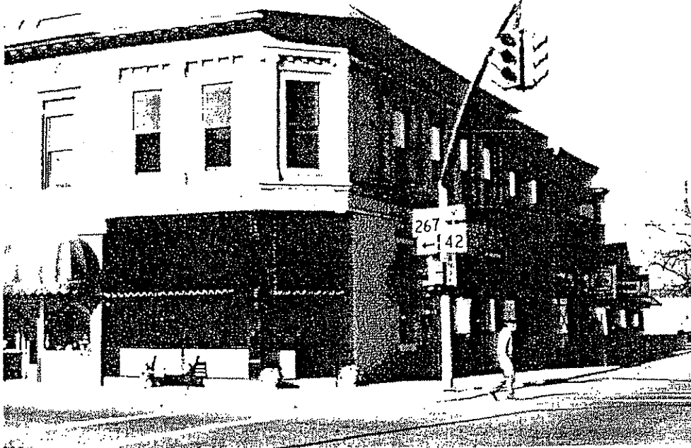
Photo 22 - Newly rehabilitated building in central business district is vacant.
