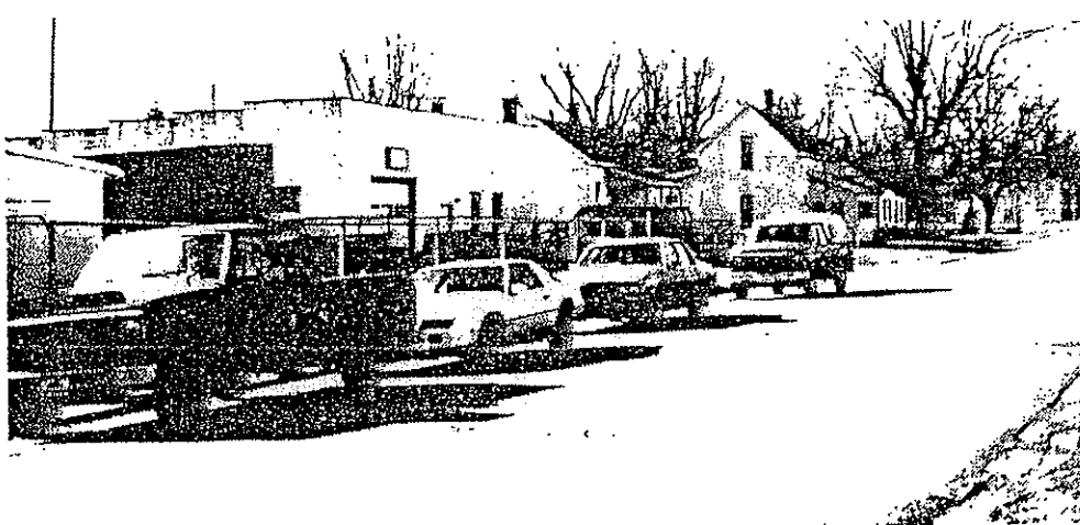
Photo 15 - Intermixture of industrial and residential uses with on-street parking due to inadequate facilities.
