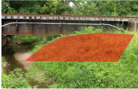
Photo 10: Accumulated Sediment Under at RR
