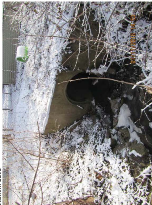
Photo 51: Upstream end of 30"RCP, west of Westwood Drive Station: 211
