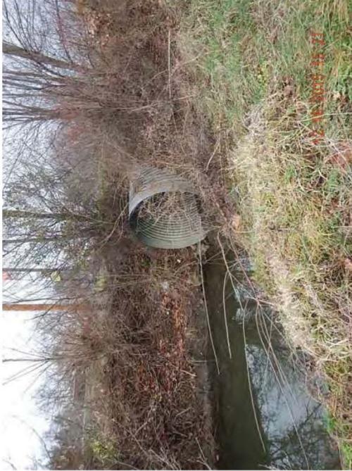
Photo 2: 9ft CMP outlet near Squealers BBQ Station: 100
