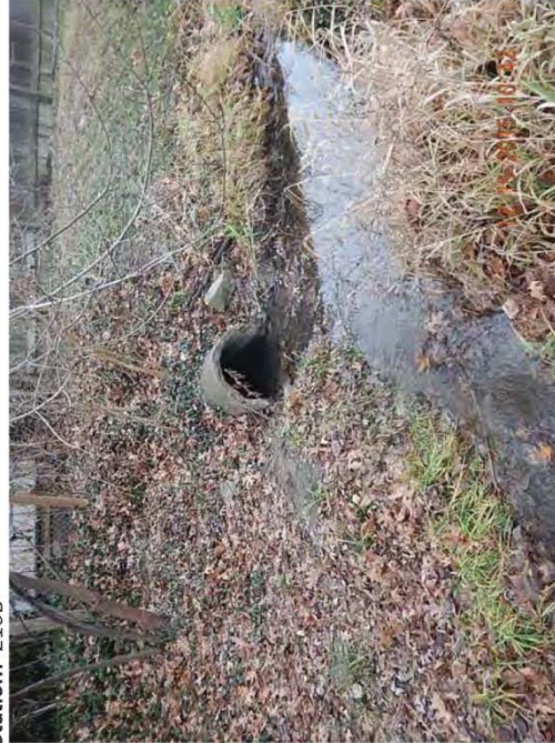
Photo 52: Outlet from Westwood drive into backyard ditch Station: 212
