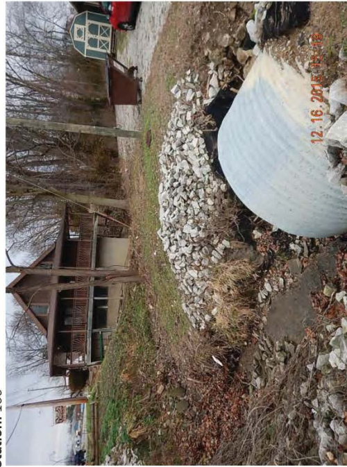
Photo 3: 9ft CMP near Squealers BBQ Station: 102
