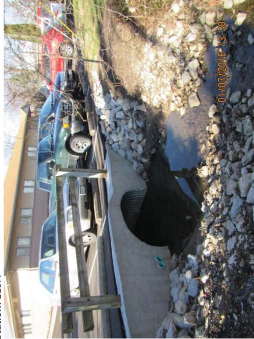
Photo 16: Culvert under Orthodontics parking lot Station: 121
