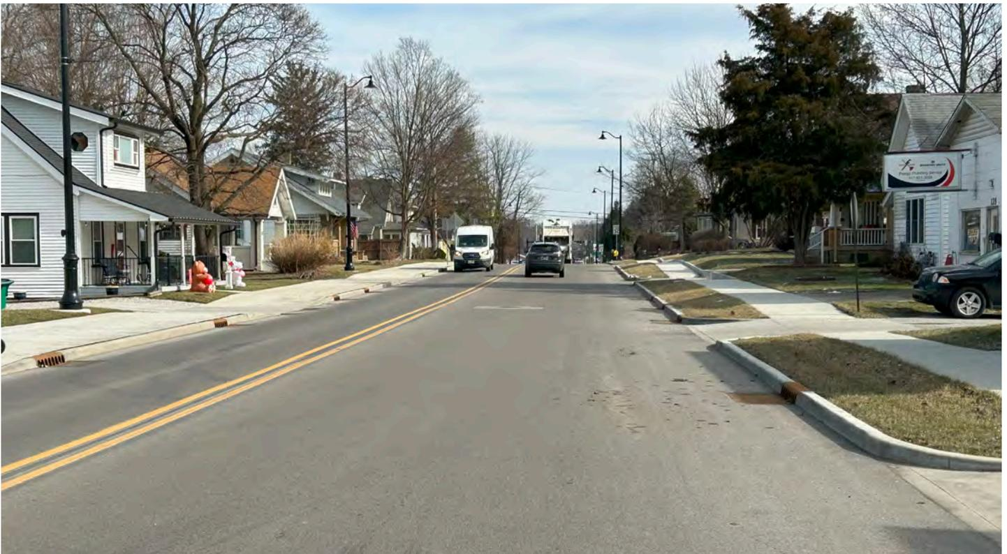
*High Street / State Road 42 was recently repaved and new sidewalks, curbs, and storm drain inlets were installed.*
